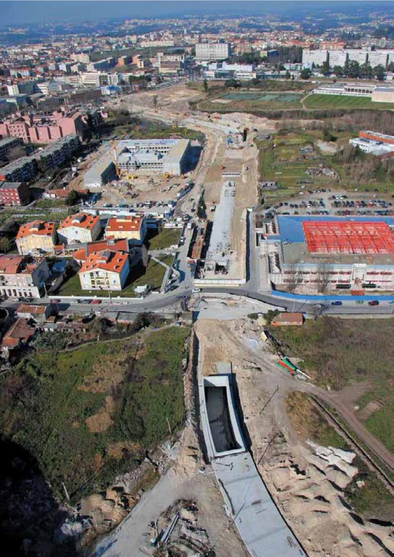
After the works to divert utilities networks, initiated in 2002, the excavation of the pit at Rua do Paraíso was initiated in March 2003. During 2004 the subsoil was excavated and the internal structures were executed. These works are expected to be completed in the first months of 2005, so that finishing works can be started.
